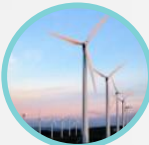
On site land-based wind generation
